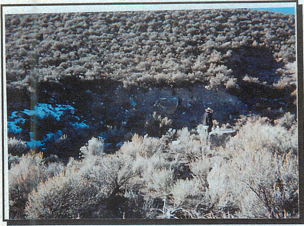
Photo No.15 Remnants of the Old Mine Tunnel Just West of the Dump Just Below the Rock Out Cropping
