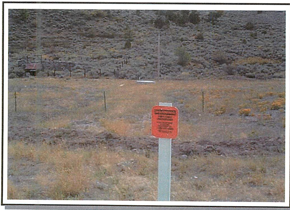
Photo No. 12 A Warning Sign for a Buried Telephone Utility Line Just South of U.S. Highway 6 on the Homansville Property
